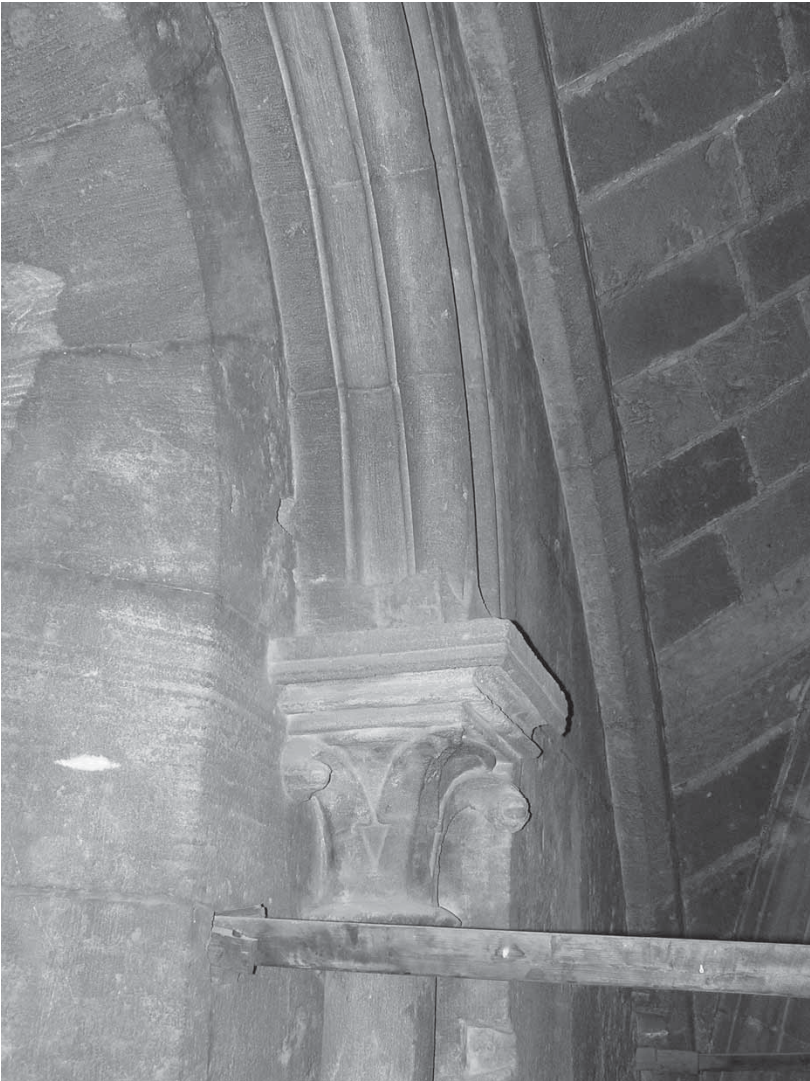
Fig. 18: Bellapais Abbey, church, west front window, detail of colonette capital and moulded arch [M. Olympios].
